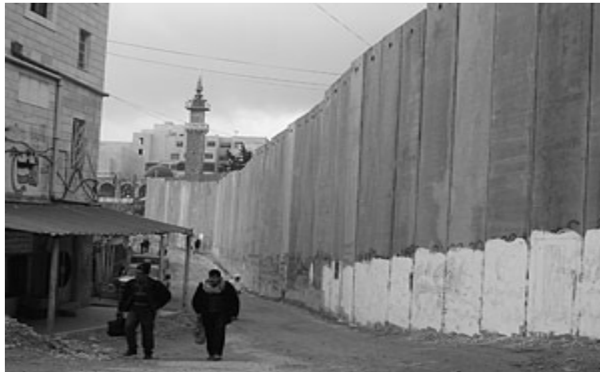
Photo 3: Nine-meter-high Wall Splitting the Palestinian Community of Abu Dis, East of the Old City of Jerusalem
