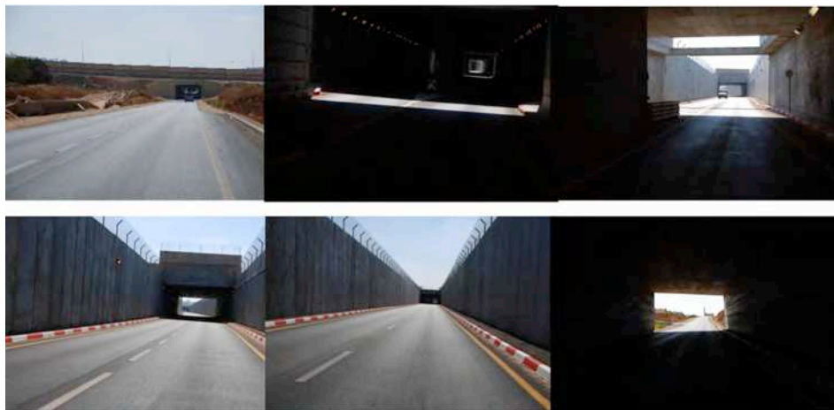
Figure 6: Bridges and interchanges shaping the fabric of life roads. (Source: Author)
