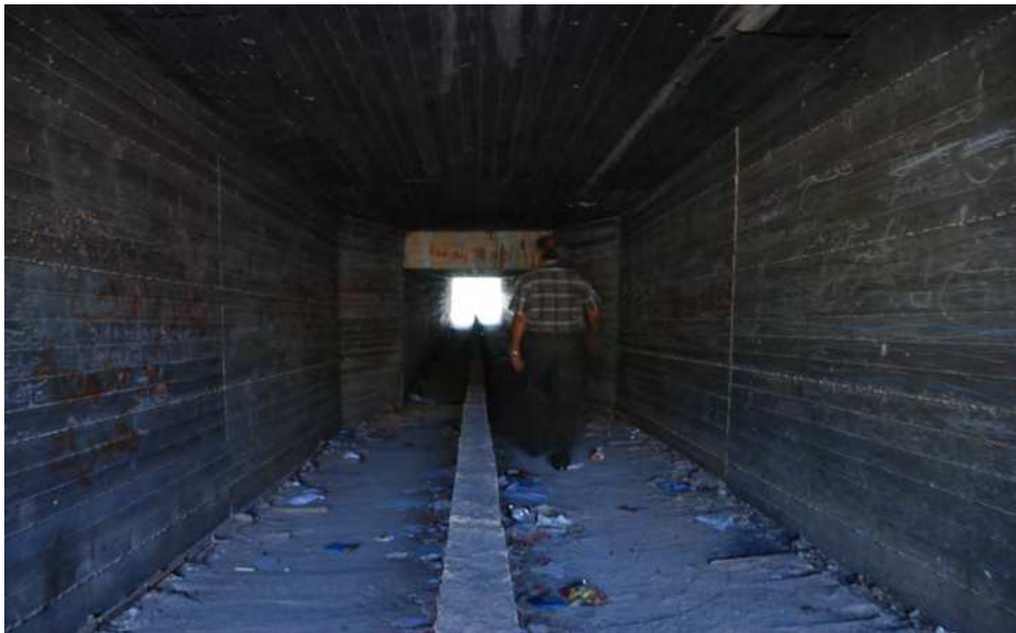
Figure 4: Viaduct for school children under Road 443. (Source: Author)
